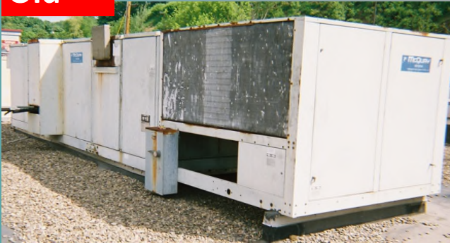
Conventional rooftop units usually do not have the moisture removal capacity needed for supermarkets
