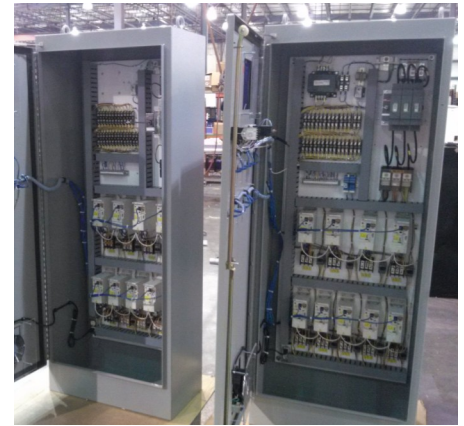
Control cabinets for 18-cell fan array.
