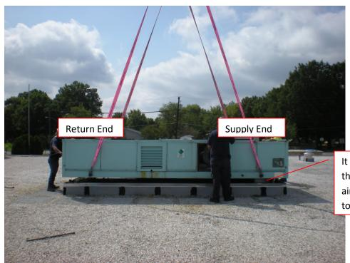
It may be difficult to tell in this picture but the supply air duct is still connected to the existing unit.
