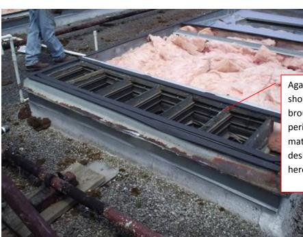
Again, a different job but this picture shows how the zone dividers are brought up level to the curb perimeter and covered in gasket material. The new S4 unit is designed to create a compression fit here.
