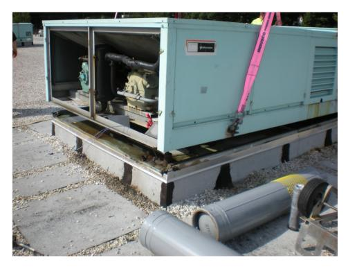
The crane should lift the old unit VERY slowly while observers are watching for wires, pipes, or connections that were missed.
