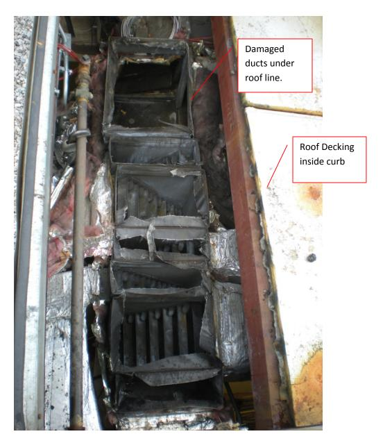
The contractor for this job evaluated the conditions and made the determination to go ahead and set the new Seasons 4 RTU without have the duct repair complete. There was enough space below the roof line and the sheet metal contractor was able to make the duct connections from underneath the roof. This is not always an option. Seasons 4 highly recommends making the necessary duct repairs before the new unit is set in place.
