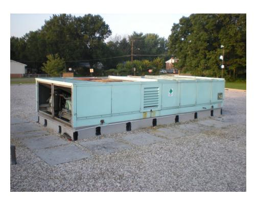
The above picture is that of a Carrier multizone roof top unit to be replaced. Before rigging the old unit for the lift, make sure that all electrical, piping, and ductwork is disconnected from the existing unit.
