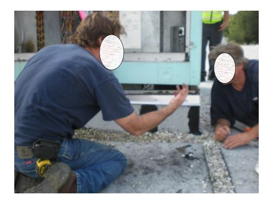
As soon as it was noticed that the supply air (SA) ductwork was still attached to the roof top unit, the lift was stopped. The contractor then took a closer look at the unit to see how the duct was attached to the RTU. In many cases, Carrier instructed the original installing contractor to screw the SA ductwork to the underside of their unit. Sometimes, the connection can be broken by a pry bar when the unit is lifted a few inches above the curb.
