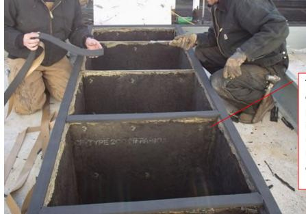
This is a different job and contractor than the previous picture. The picture shows the installing contractor placing the new gasket material provided by S4 onto the supply air duct dividers and perimeter.
