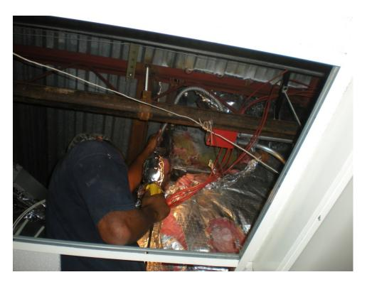
Above, a worker disconnects the supply air duct drop loose from the existing ductwork.
