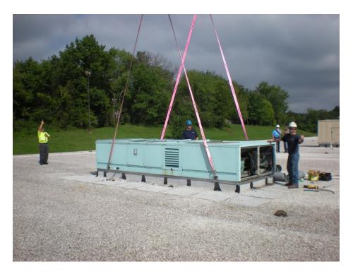
Seasons 4 recommends using spreader bars with straps or chains to lift the old unit out of place. If spreader bars are not available, straps that are 40' in length are acceptable.
