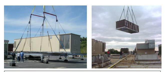
IF SPREADER BARS ARE USED, THEY MUST BE 4 FEET WIDER THAN THE UNIT. IF STRAPS ARE USED, THEY MUST BE AT LEAST 40 FEET LONG.
