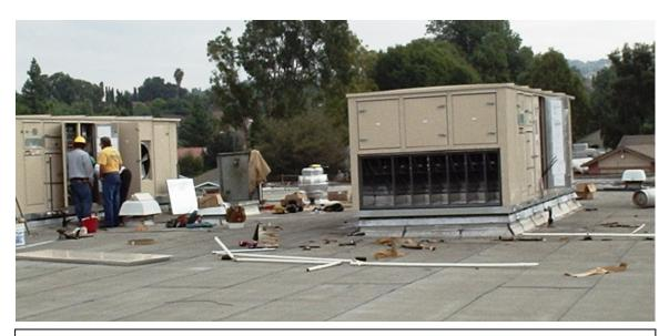
REMOVE THE RIGGING AND REPLACE THE END ZONE PANEL. CAULK THE END PANELTO ASSURE A WEATHER-TIGHT SEAL. CONNECT THE POWER, CONTROLS, GAS (IF APPLICABLE) CONNECTIONS.
