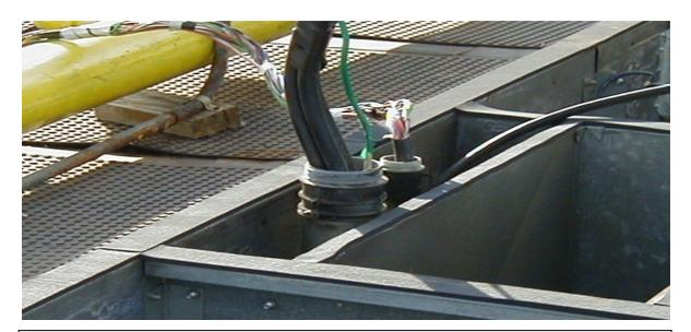
PREPARE THE UTILITY CONNECTIONS AND POWER WIRES TO INSERT THROUGH THE NEW UNIT POWER CHASE.
