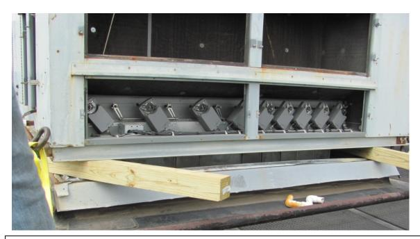
MAKE SURE THE EXISTING DUCTWORK OR THE CURB IS NOT ATTACHED TO THE UNIT.
