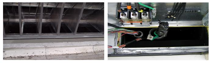
PROCEED WITH LOWERING THE UNIT INTO PLACE. CHECK DUCT ALIGNMENT AND POWER CONNECTION ALIGNMENT. MAKE ADJUSTMENTS TO ASSURE PROPER SEALING OF THE DUCTS TO THE UNIT. ALL CHASES MUST BE CAPPED AND SEALED BEFORE START-UP.
