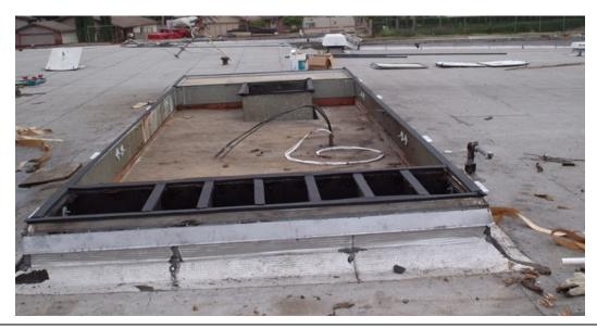
THE SUPPLY AND RETURN DUCTS MUST BE LEVEL AND SECURED TO THE TOP OF THE CURB IN THEIR ORIGINAL LOCATIONS. PROVIDE TWO LAYERS OF GASKET ON SUPPLY (EACH ZONE) AND RETURN DUCT OPENINGS, AND ONE LAYER ON THE CRUB PERIMETER TO SEAL THE CURB TO THE BOTTOM OF THE UNIT.
