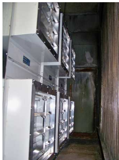
Fan cells installation in 40 years old existing unit.
