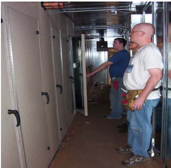
Service corridor with hinged access doors, single door handle with multiple latches, aluminum tread plate floor, exhaust fan and electric heater.
