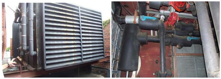
One of the existing units (AHU-4) is a 30,000 CFM multi-zone unit with a run-around loop energy recovery system with pumps and many water valves. A maintenance system nightmare. The university was looking for a more efficient ERU system with less headaches that would still match the existing curb..
