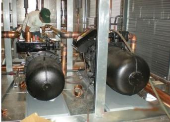
Three (3) Copeland screw compressors each with independent refrigeration circuits, air cooled condensing section, and R-134A refrigerant.
