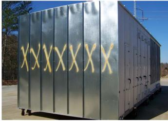
The exterior panels are fabricated from Kynar painted aluminum (never rusts). Marine-type service lights are provided in each accessible section. The unit is completely tested then split in two sections and shipped to the jobsite.
