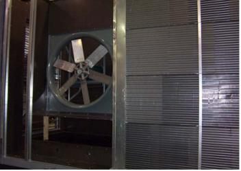
Direct drive supply air blowers with shaft grounding kits, premium efficiency motors, 2" spring isolators with Zone-4 seismic tie downs, and direct drive propeller exhaust fans are some of the requirements of the project.
