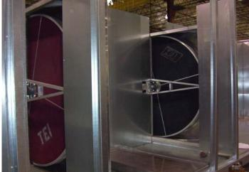
11,000 cfm of outside air at 95/77.7 deg F is conditioned thru an enthalpy wheel, dehumidified with DX coils and reheated with a sensible heat wheel to 72.3/65.3 deg F.
