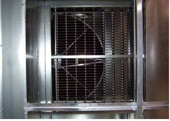
The units include Loren Cook plenum airfoil supply and exhaust air blowers, TEFC premium efficiency motors and perforated liners for sound attenuation. 70 to 85 KW auxiliary electric heat, lights in all accessible sections, 2" pleated and 12" cartridge final filters are some of the features provided with the units.
