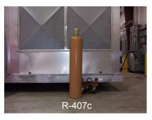
R-407c is a blend of R-32 (23%), R-125 (25%) and R-134A (52%). It can be dropped in an existing R-22 system, compressors require POE oil. It has a minimum of 8 deg F glide and about 5% to 6% performance loss.
