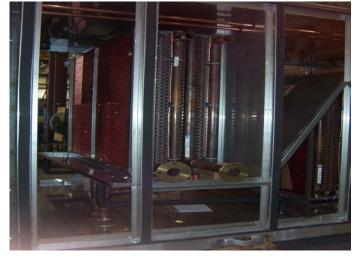
Two sets of 6-row coils with copper fins and copper tubes and stainless steel casings, along with an expansion tank and circulation pump, comprise a run-around loop that pre-cools and re-heats air up to 55 deg F leaving air temperature.
