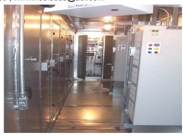
The exterior panels are embossed painted aluminum. All units are provided with service corridor and a porch with accessory stairs, service light and a switch for each section, VFD on supply and the exhaust blowers, 2" pre-filters and 12" 85% cartridge filters, and airflow measuring stations.
