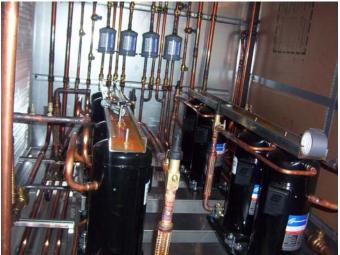
Condensing sections are provided with SWSI airfoil plenum blowers with VFD, scroll compressors with sound blankets and acoustical lovers for low sound levels, 407c refrigerant, lead/lag compressor rotation and hot gas bypass on all circuits.
