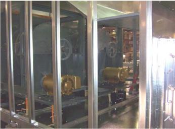
Each unit consist of two supply and two return air blowers with back draft damper, 100 HP premium efficiency supply and 25 HP return air motors for 100% redundancy.
