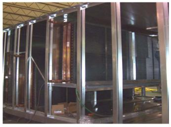
There are 4 chilled water coils and 4 hot water coils with stainless steel casing in each unit, the headers are stubbed out of both sides of the units for ease of coils removal from each side.
