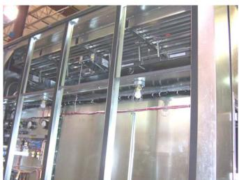
End return, top discharge with supply and return smoke dampers, outside air monitoring station and outside air and return air aluminum airfoil dampers.
