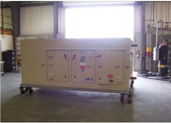
2" double wall panels with embossed painted (Pueblo tan) aluminum exterior with single door handles and labeled sections and doors. The units are ETL listed.
