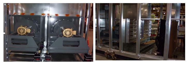
Two direct drive airfoil SWSI plenum blowers are provided with premium efficiency motors and VFD'S. The blowers are also provided with 2" seismic spring isolators and blower isolation dampers. Each fan is designed to provide 75% of the total airflow.
