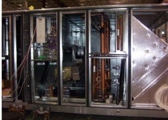
The first section consists of condenser coils, condenser fans, two 40 ton Copeland Discus compressors, dual airfoil SWSI blowers with two blower motors, DX cooling coil, hot water heating coil and 140" long multi-zone damper and actuators. The second section includes return air opening, economizer section, and filters.
