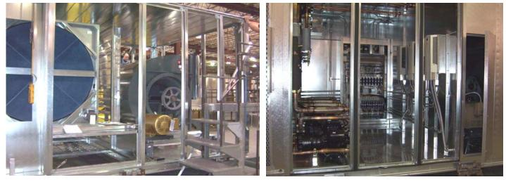
An airfoil DWDI housed exhaust fan with a 60 horsepower premium efficiency motor and a VFD will exhaust 62,910 CFM from the building.
