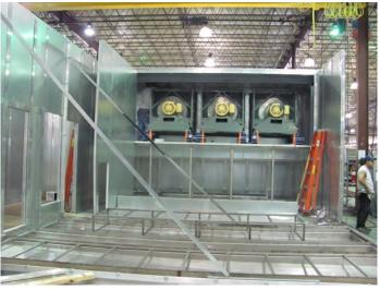
Multiple direct drive supply and exhaust air blowers with premium efficiency motors, fan isolation dampers and trolley rails for motor removal are some of the features provided.
