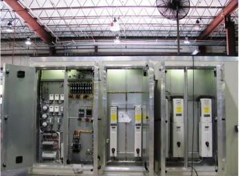
AHU-1 is provided with a walk-in service corridor. All motors are driven with ABB drives. DDC controls are provided and programmed by Powers of Arkansas and installed by Seasons-4.
