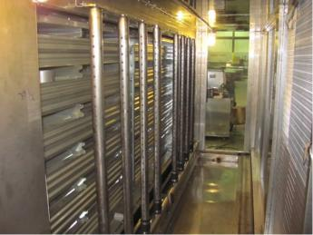
Chilled water cooling coils, integral face and bypass heating coils, humidifier, service lights, UV lights, smoke/fire dampers, and high efficiency filters are additional features.
