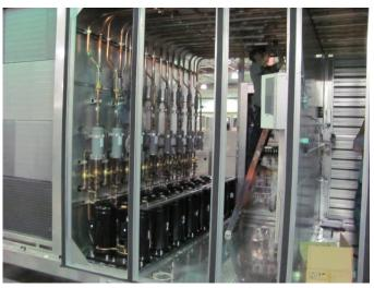
16 scroll compressors with a digital lead compressor mounted in a walk-in service vestibule with aluminum tread plate floor, vestibule exhaust fan and electric heater.
