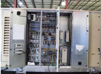
Heatco tubular gas burners, airfoil plenum blowers, premium efficiency blower motors, ABB drives, UV lights, HEPA filters, airflow measuring stations and DDC controls are some of the features provided.
