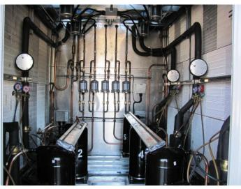
There are a total of five (5) scroll compressors, two of the compressors have digital capability (10 to1 modulation). The air cooled condensing section is design for 105 deg F ambient with R-410a refrigerant.
