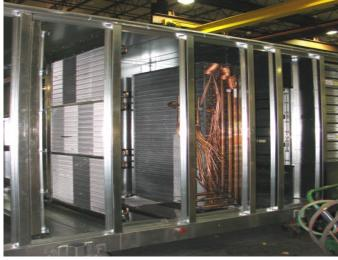
The unit consist of two paths (two air streams), outside air path and the return air path. Each path has its own independent compressors, condenser coils, evaporator coils and sub-cool reheat coils. A hot gas re-heat coil is installed down stream of the mixing plenum for re-heat when needed. Both paths condition the air down to 41 deg dew point.
