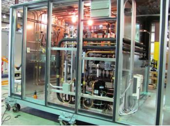
Each circuit has Copeland scroll compressors with a digital lead and water cooled condensers located in a walk-in service vestibule with aluminum tread plate floors and electric heaters.
