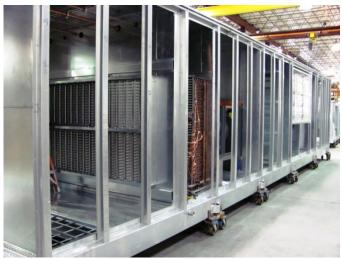
Energy recovery wheels, open resistance electric heaters, airflow monitoring stations, CO2 sensors, security dampers, recirculation condensation pump and DDC controls are additional features.
