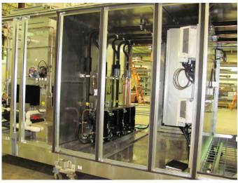
Welded galvanized steel base and the floor, evaporative cooled condensing sections, scroll compressors with a digital lead compressor, walk-in service vestibule with welded aluminum tread-plate floor are some of the features of these units.
