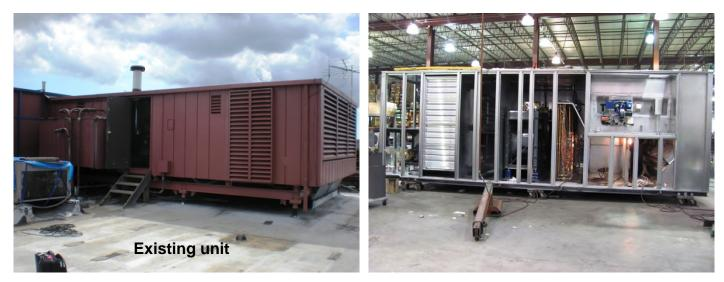
The existing unit is steel mounted with split condensing section. The new custom direct replacement unit will match the existing steel, supply and return air openings, power supplies (there are 6 power supplies), and gas connection.
