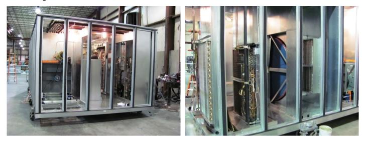
Walk-in service corridor for ease of accessibility and maintenance, service lights, hot gas reheat coils, 2" foam insulated panels with R value of 13 are some of the features provided.
