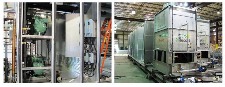
The cooling system is provided with 2 screw compressors and evaporative condensing sections with R-134a refrigerant. The compressors, control panel and VFDS are mounted in a walk-in service vestibule with aluminum tread plate floor.
