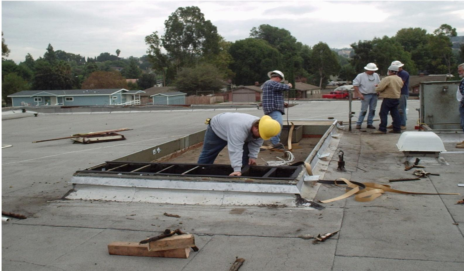
**The existing unit curb is cleaned and covered with factory provided gasket.**
